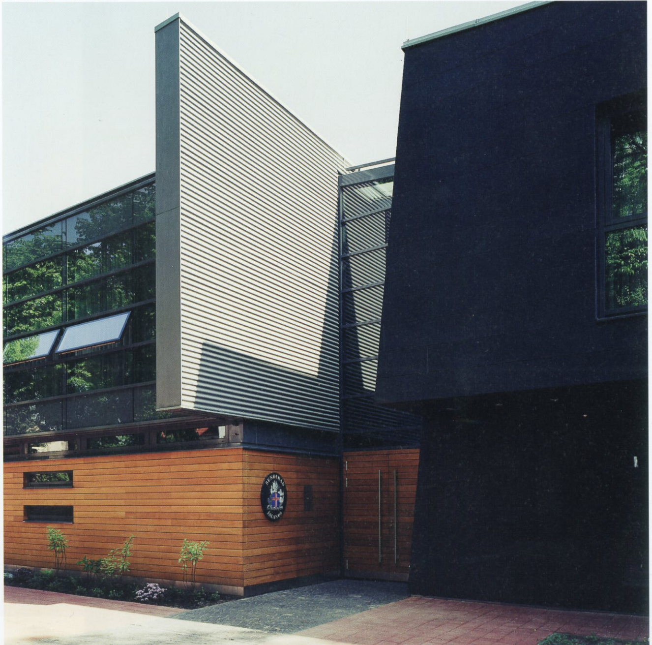
The main entrance in glass, corrugated zinc plate, black stone and oak. The cleft that divides the building into two parts alludes to the Icelandic landscape.
