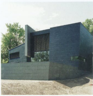
Typically Icelandic mountain formations and waterfalls have inspired the south façade of stone and glass.
